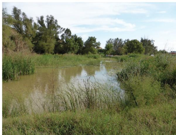
Fig. 5. Free water surface constructed wetland for treatment of agricultural drainage planted with *Phragmites australis*. Laluzea, Spain
