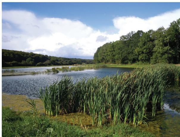
Fig. 4. Free water surface constructed wetland for treatment of tile drainage planted with *Typha latifolia* at Rodstenseje, Denmark
