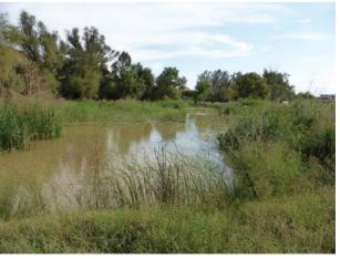
Fig. 5. Free water surface constructed wetland for treatment of agricultural drainage planted with *Phragmites australis*. Laluzea, Spain Photo: author
