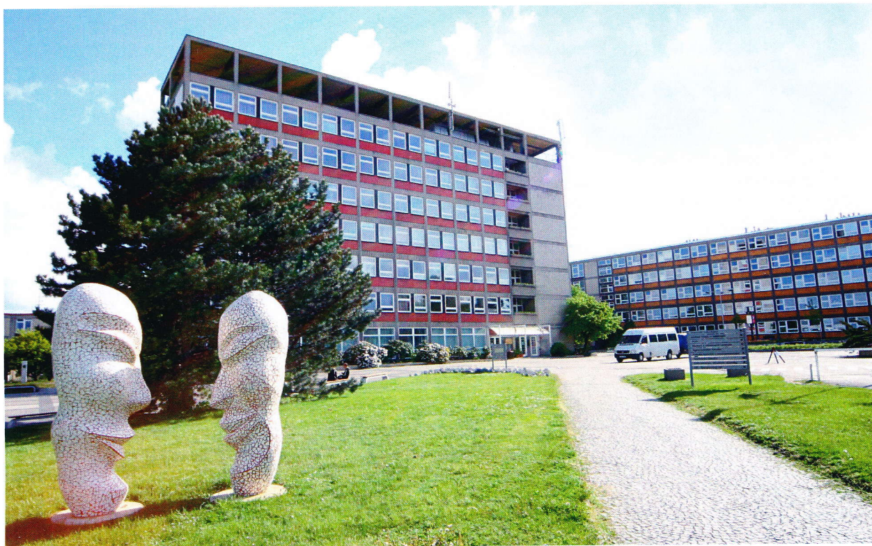
The campus of the Czech University of Agriculture in Prague-Suchdol was built in 1953–1956
